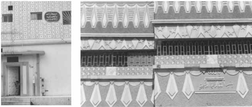
Fig. 1.34. Attempts by inhabitants of the transitional house in the 1970's to decorate their house façades (their attempts appeared when concrete became the only material for construction). Source: Author.
